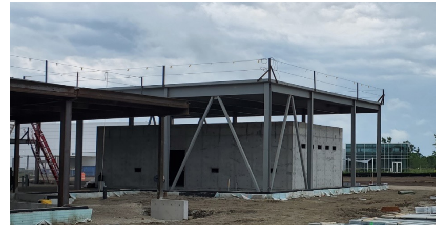
Concrete ISN enclosure walls and roof complete
