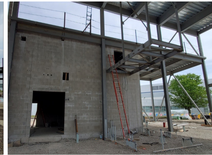
AML masonry walls with the catwalk to HEXM
