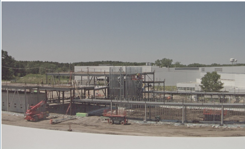
Site Photo from June 30, 2021
