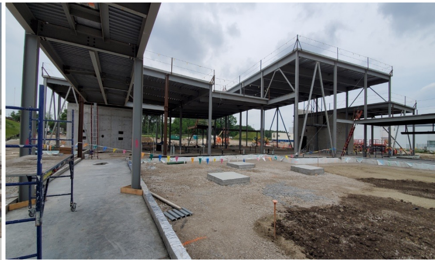
Steel Structure of the LBB and the corridors
