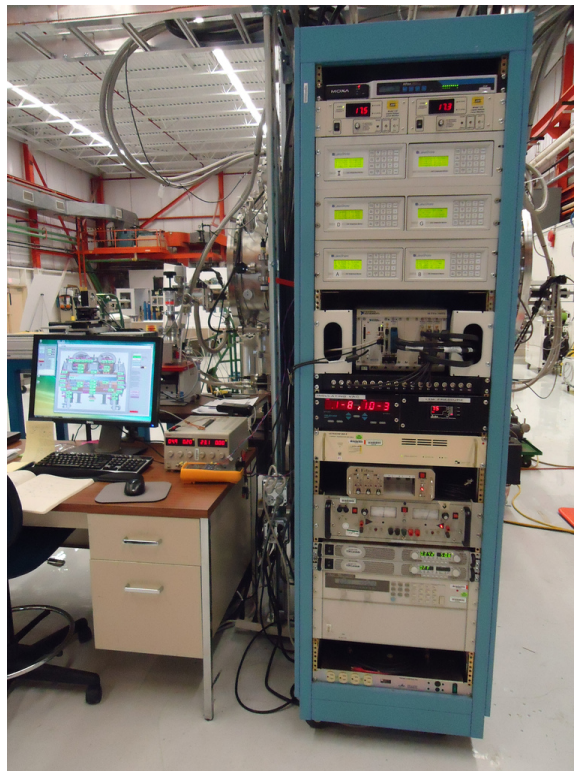
Figure 3.5-22: Control system rack with all components installed.
