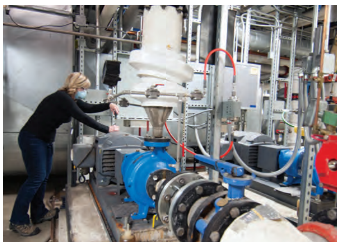
Debra Curry, AES Mechanical Operations and Maintenance Group Technician Senior: “One of my tasks is to twice a month record and document vibration and temperature readings from multiple Gould and SPX accelerator-system pumps. These recordings are then analyzed to determine what pumps are failing or near failing, to subsequently be rebuilt or replaced.”
