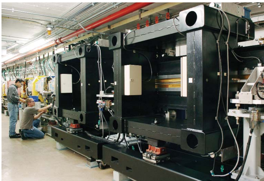
Hahn Bui (left) and Adam Brill (right), both ASD, checking diagnostics near the canted undulators at sector 23.
